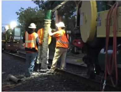
Potholing for Utilities
