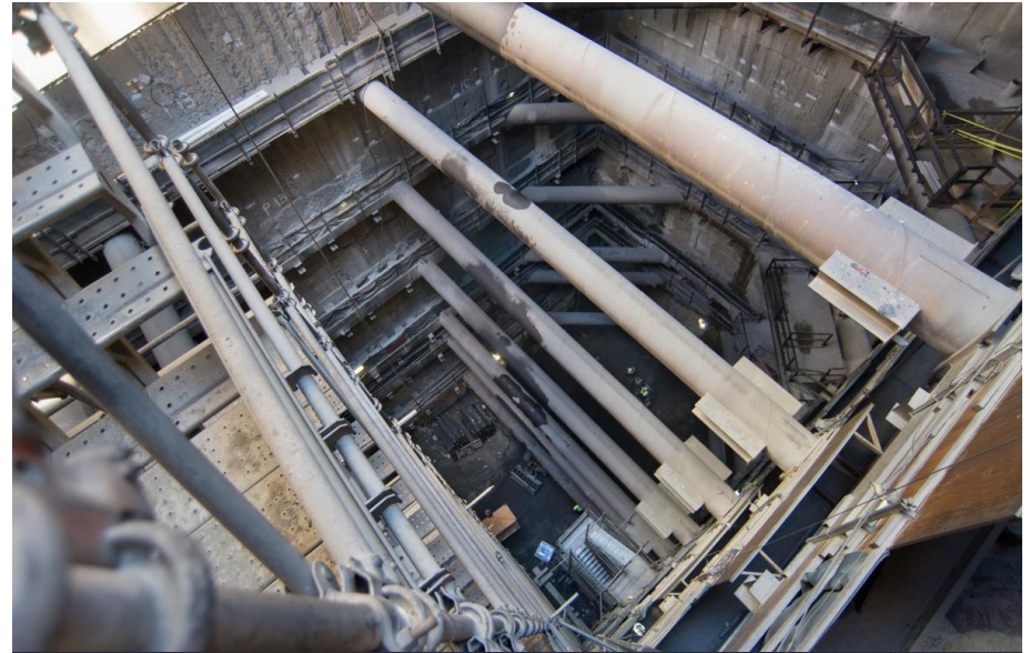
View looking down into the station headhouse
