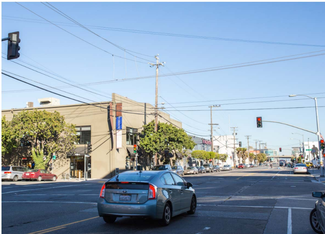
Mast Arm Signal
