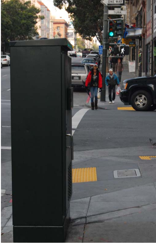
Traffic Controller and new curb ramps
