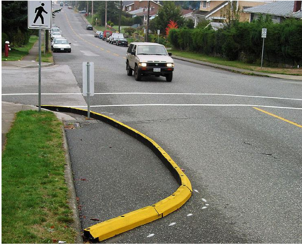
Figure A3-13 Curb Extension using Temporary Materials
