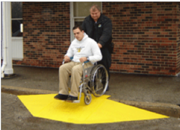
FIGURE 2-25. TEMPORARY CURB RAMP
