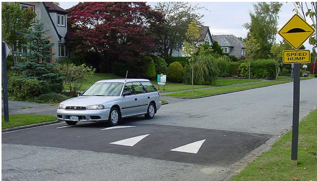
Figure A3-9 Concrete Speed Humps
