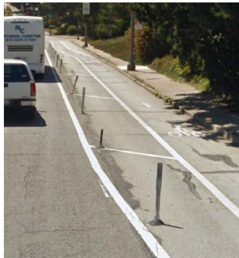
Existing Conditions: Portola Drive
