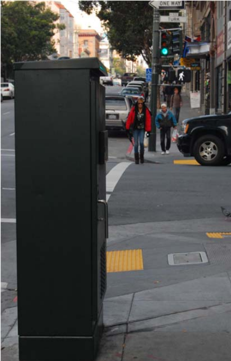
Traffic Controller and new curb ramps
