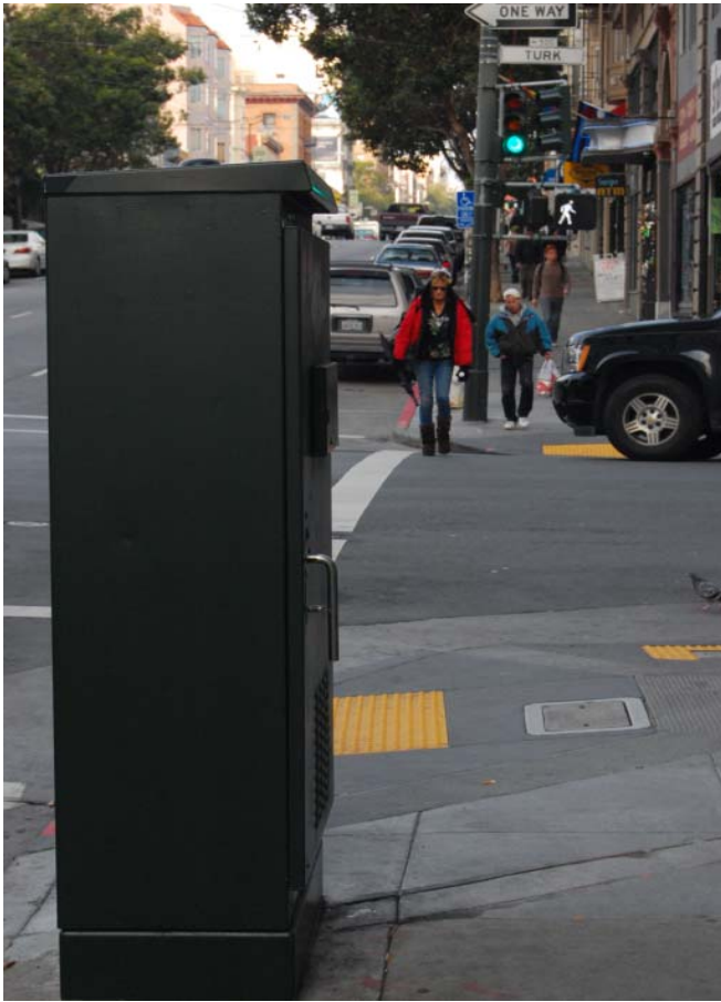
Traffic Controller and new curb ramps
