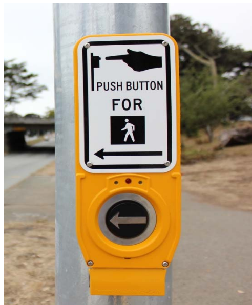
Accessible Pedestrian Signals
