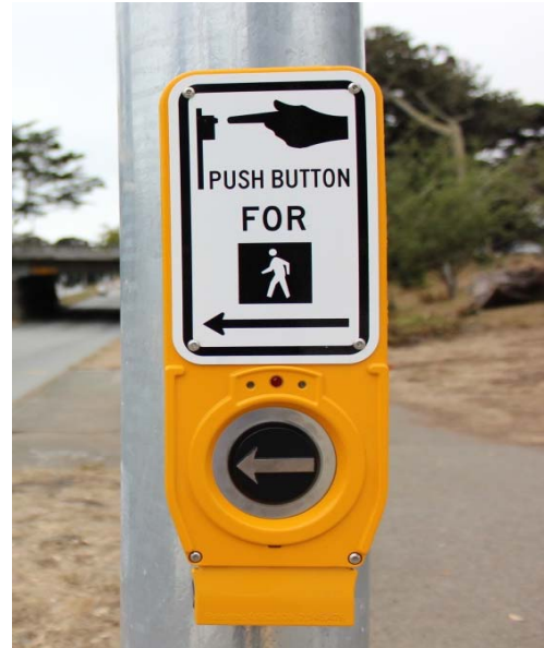
Accessible Pedestrian Signals
