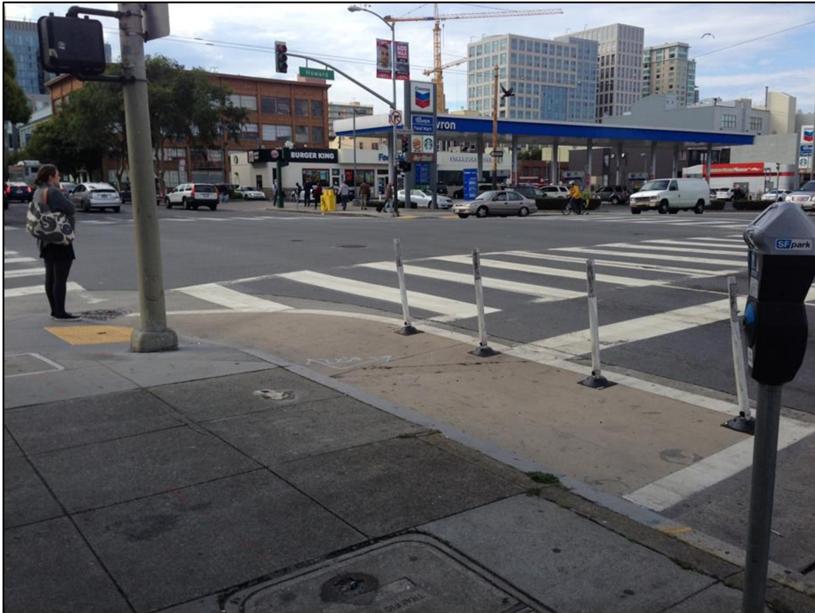
Example of a painted safety zone
