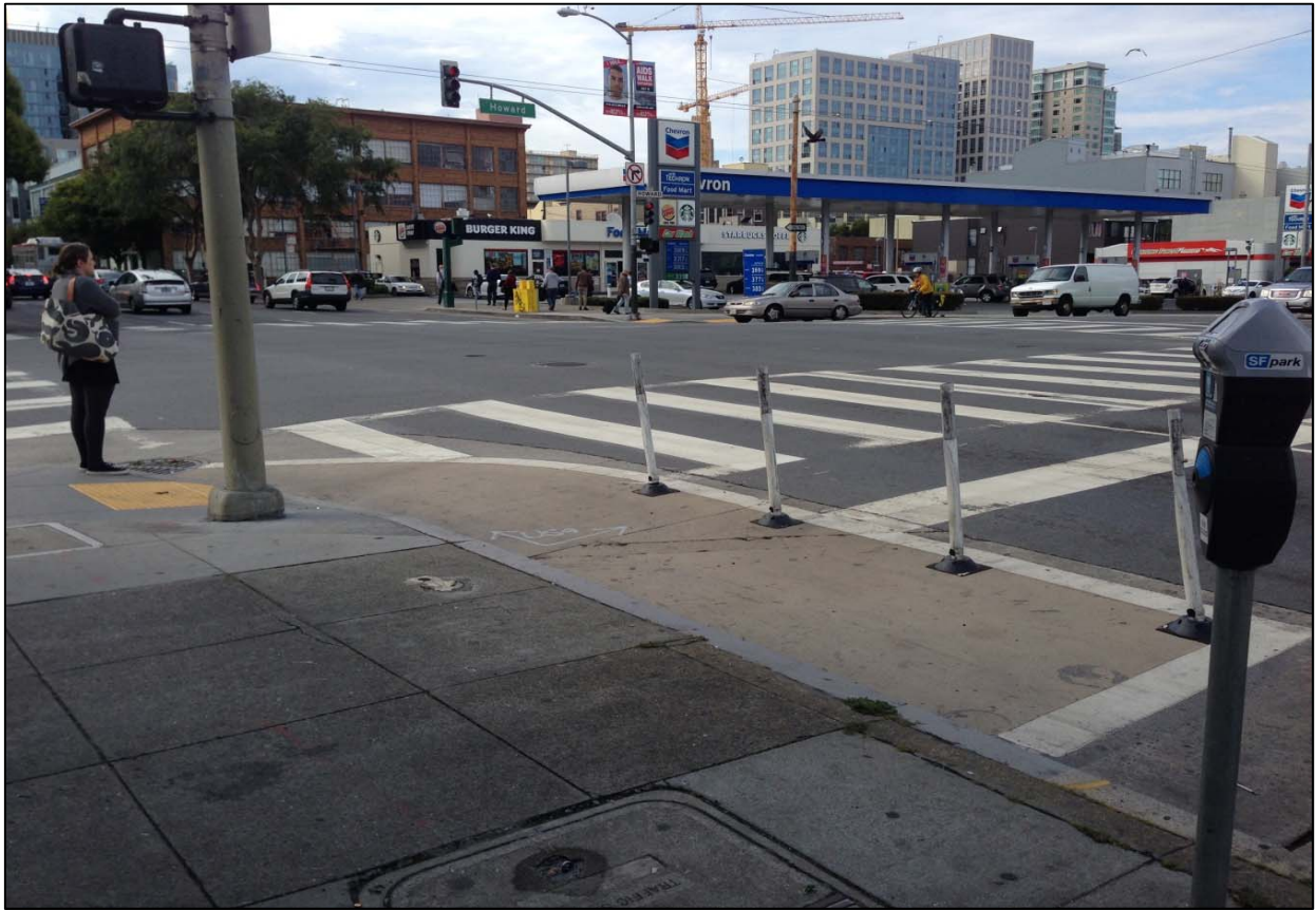
Figure 3. Example of a Painted Safety Zone (PSZ) at Howard Street in San Francisco.
