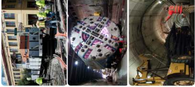
IMPLEMENTATION Planning, Design, & Construction
