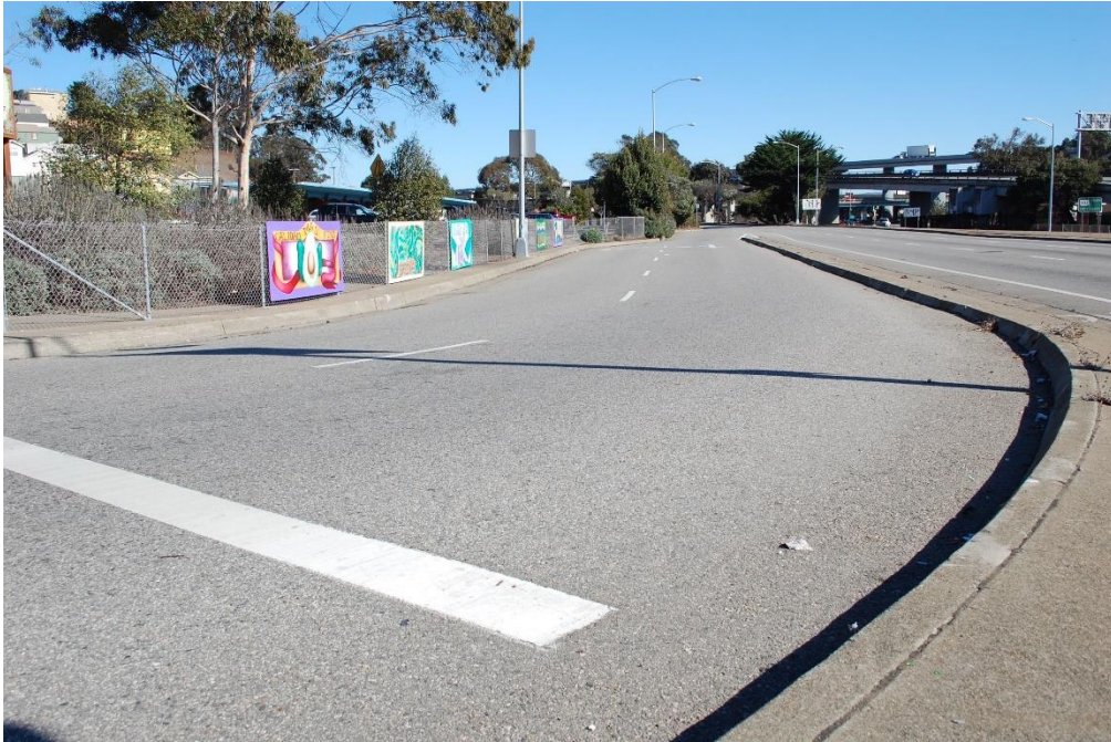
Figure 1: Alemany Westbound and Putnam Street
