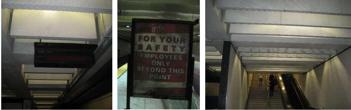
Figure 3: Examples of Acoustic Panels, Lack of Cleanliness
