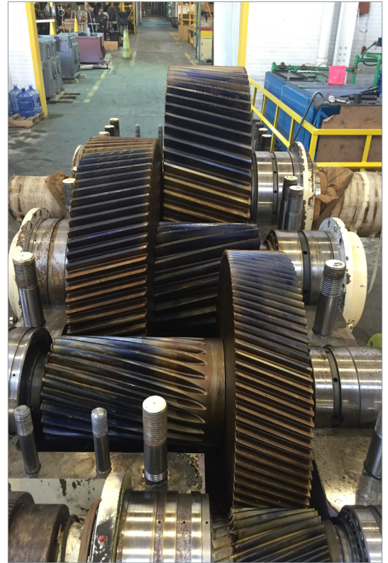
▲ Local half-cent transportation sales tax funds supported the cable car gearbox rebuild.
