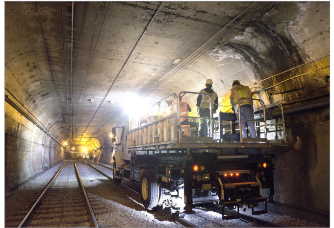
▲ Crews Installing brackets to carry communications cables in Twin Peaks Tunnel.
