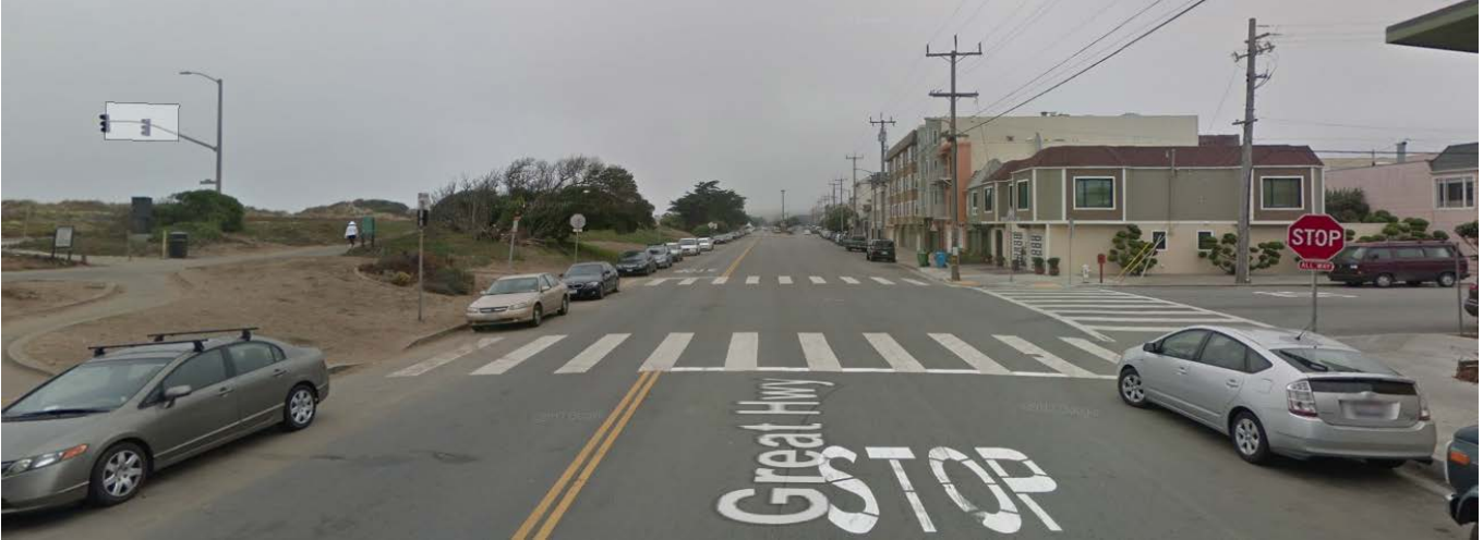
Existing conditions: Lawton Street
