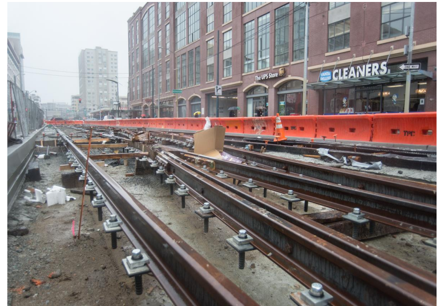
Rain falls in SoMa at a double track crossover installed on 4 th Street between Townsend and Bluxome
