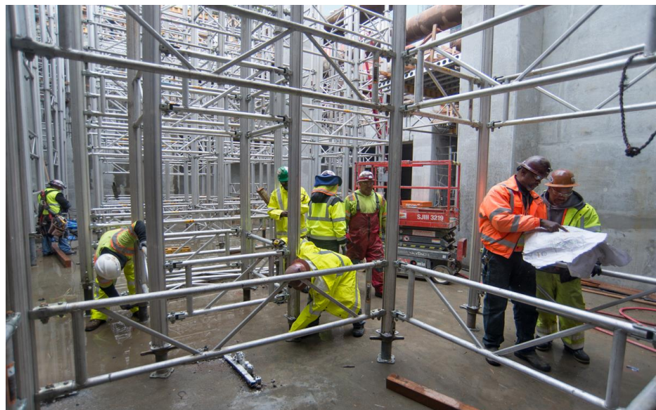
Large sections of scaffolding are being positioned inside the station headhouse to hold up future roof deck concrete forms
