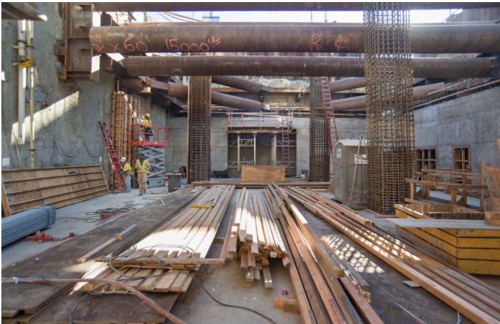
Yerba Buena/Moscone Station: Interior walls and the Mezzanine-level floor slab are being constructed inside the station headhouse.
