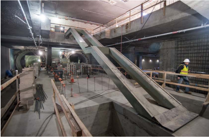
Yerba Buena/Moscone Station: Steel framing for stairs and escalator components are being installed inside the station box under 4th Street.
