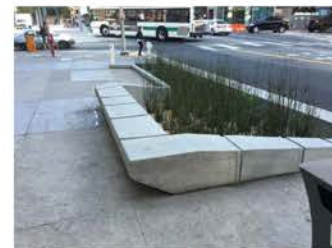
Bulbouts with raingardens help capture and treat stormwater, and can provide seating and other landscaping / habitat opportunities
