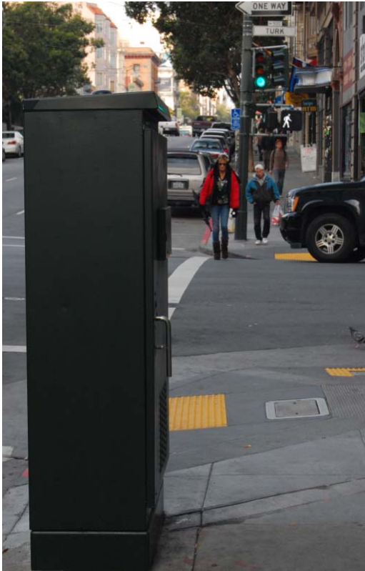
Traffic Controller and new curb ramps
