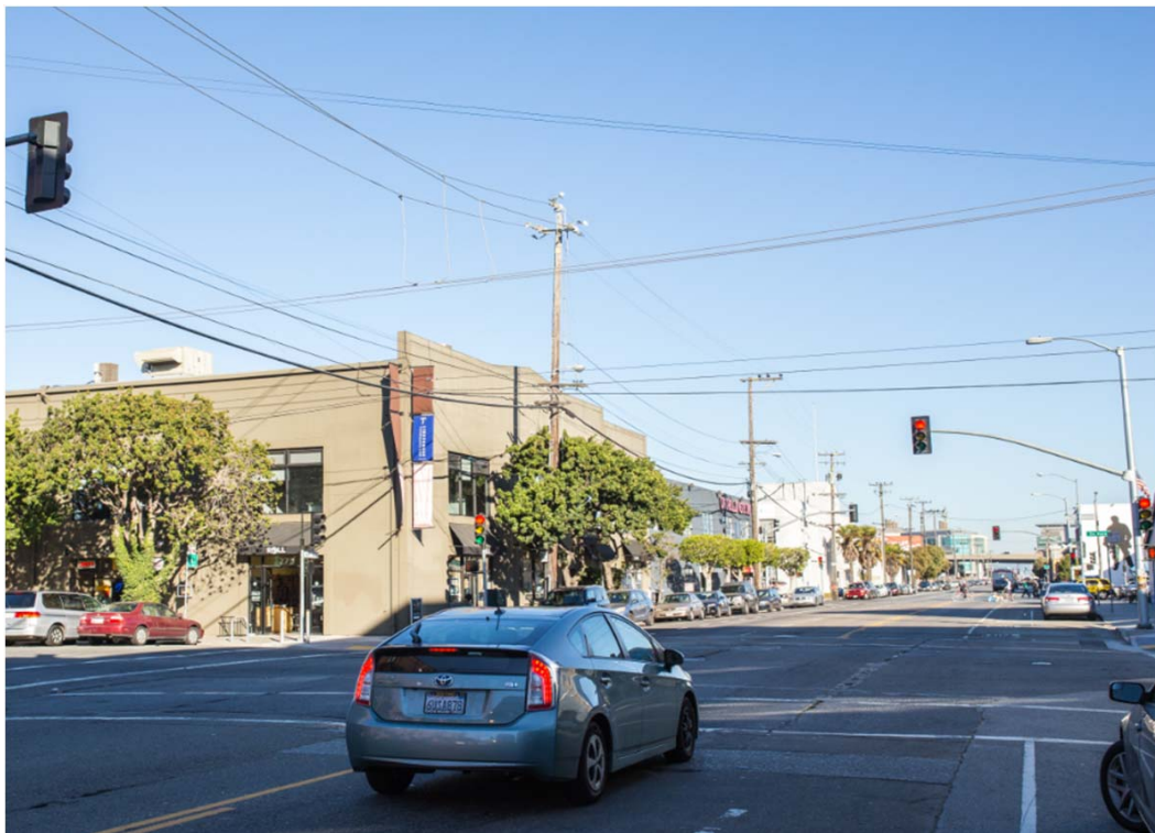
Mast Arm Signal
