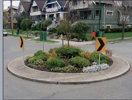
Comprehensive, long-term improvements at high injury corridor locations, determined through WalkFirst analysis
