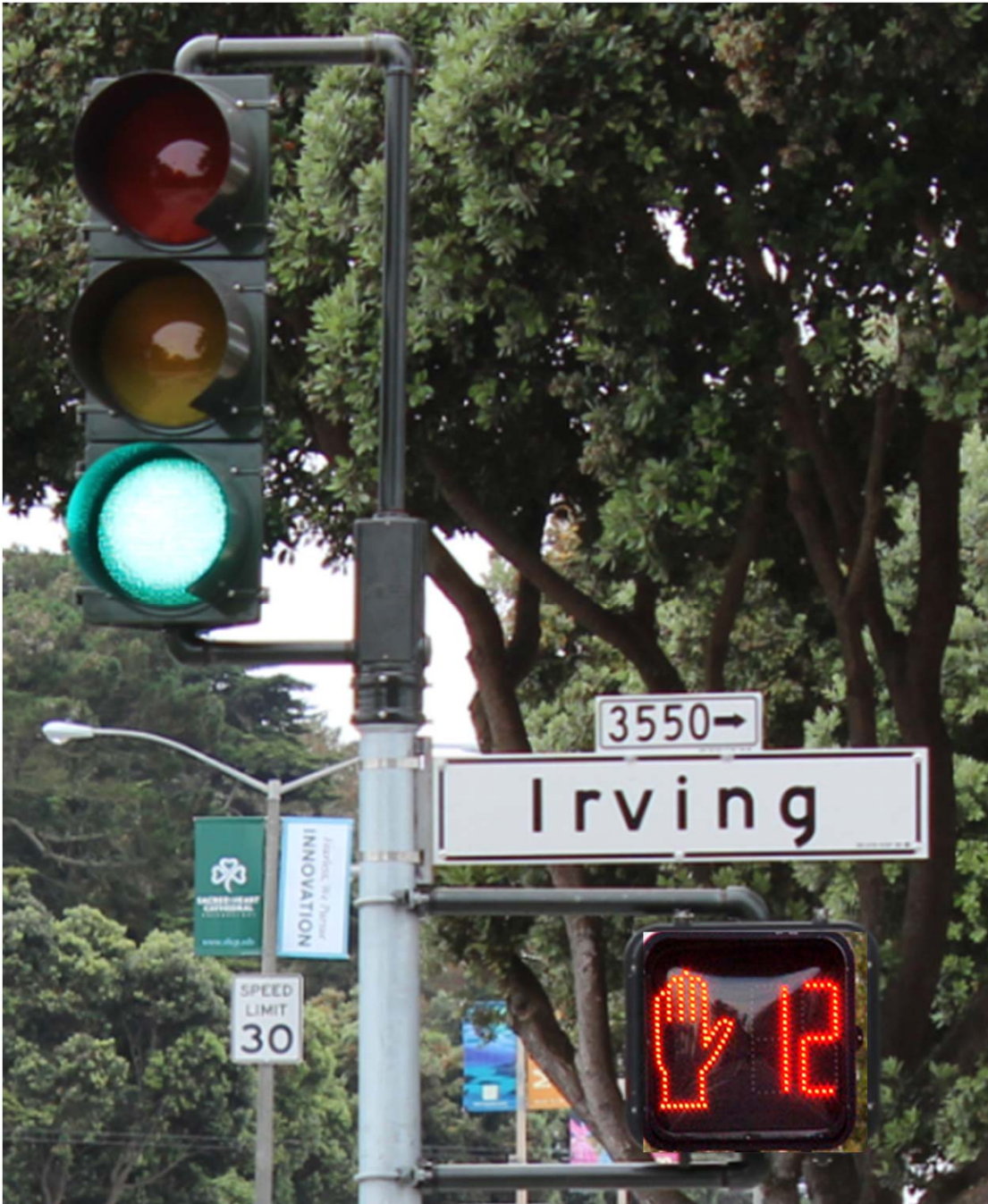
New 12-Inch Vehicle Signal with New Pedestrian Countdown Signal
