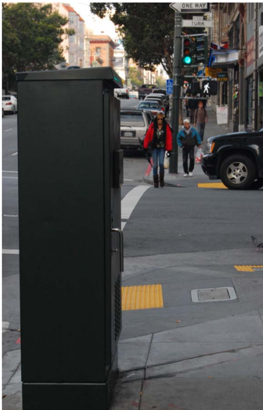
Traffic Controller and new curb ramps
