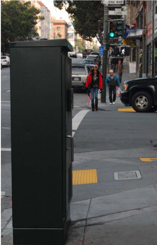
Traffic Controller and new curb ramps
