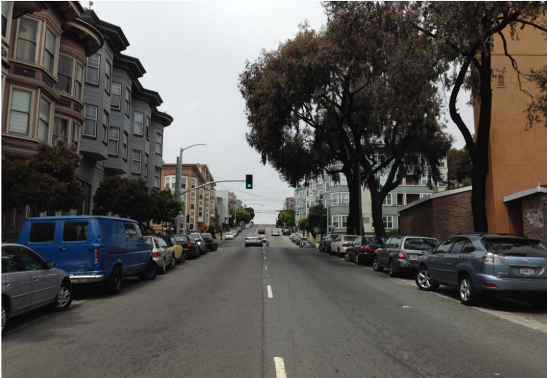
Mast Arm Signal
