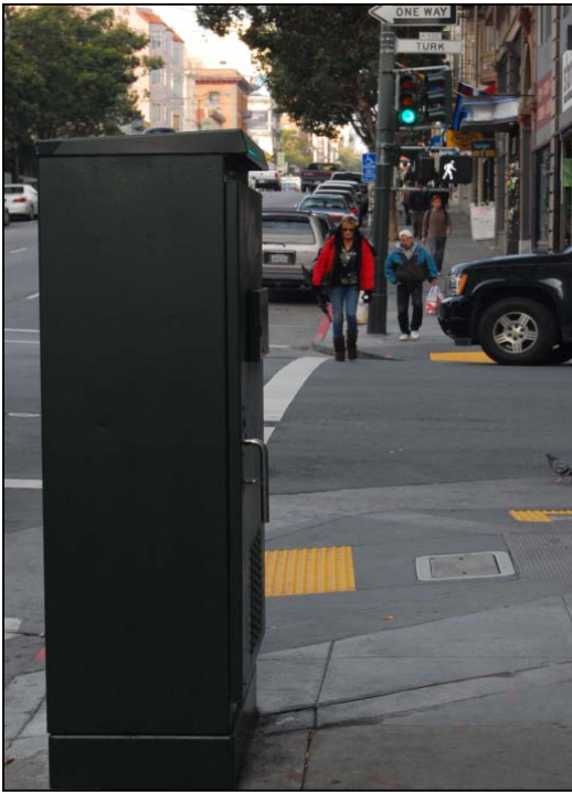
Traffic Controller and new curb ramps
