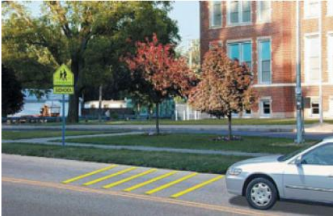
Figure A3-6 Rumble Strips
