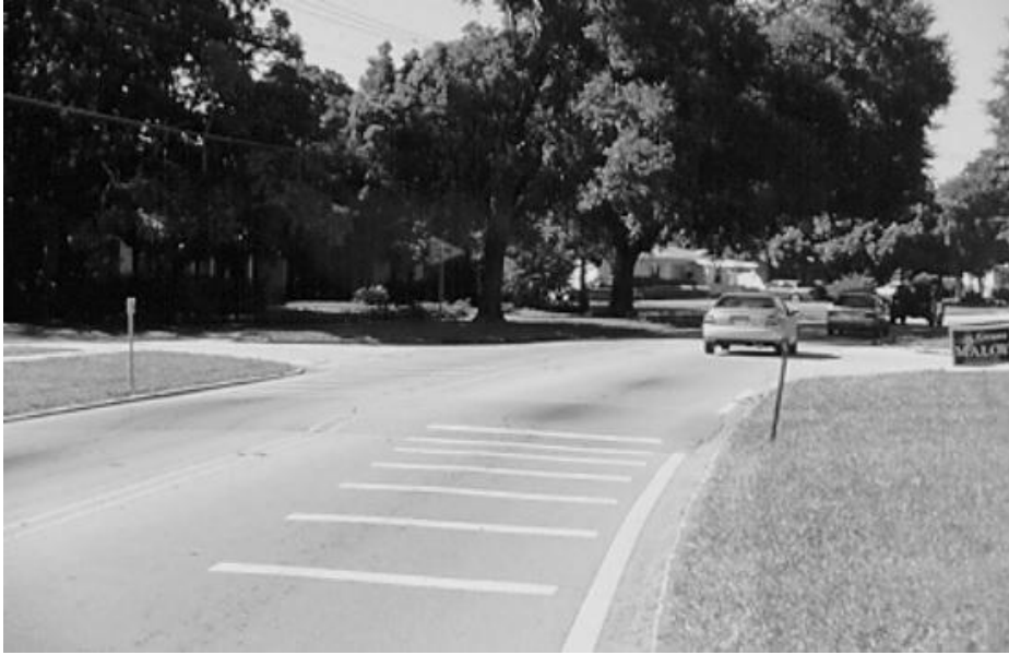
Figure A3-7 Transverse Marking
