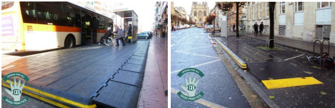
Figure A3-14 Zicla Bus Boarder – Curb Extension
