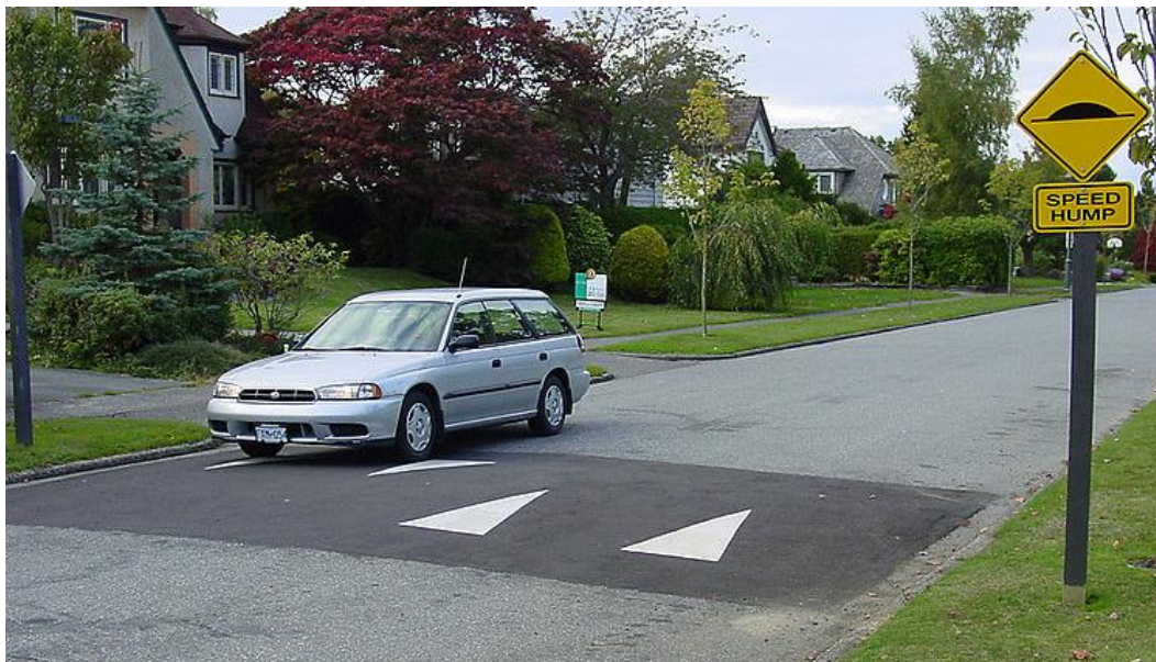
Figure A3-9 Concrete Speed Humps
