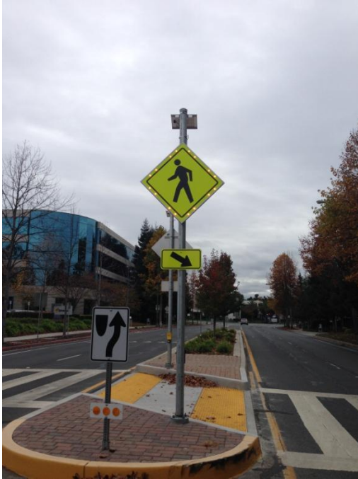
Figure A3-4 Beacons Embedded in Signs
