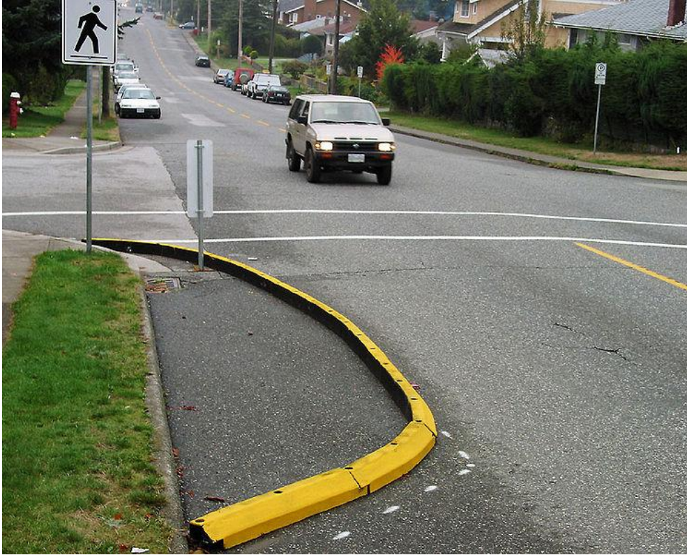
Figure A3-13 Curb Extension using Temporary Materials
