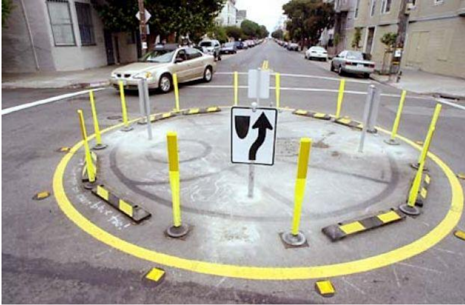
Figure A3-12 Roundabout using Temporary Materials
