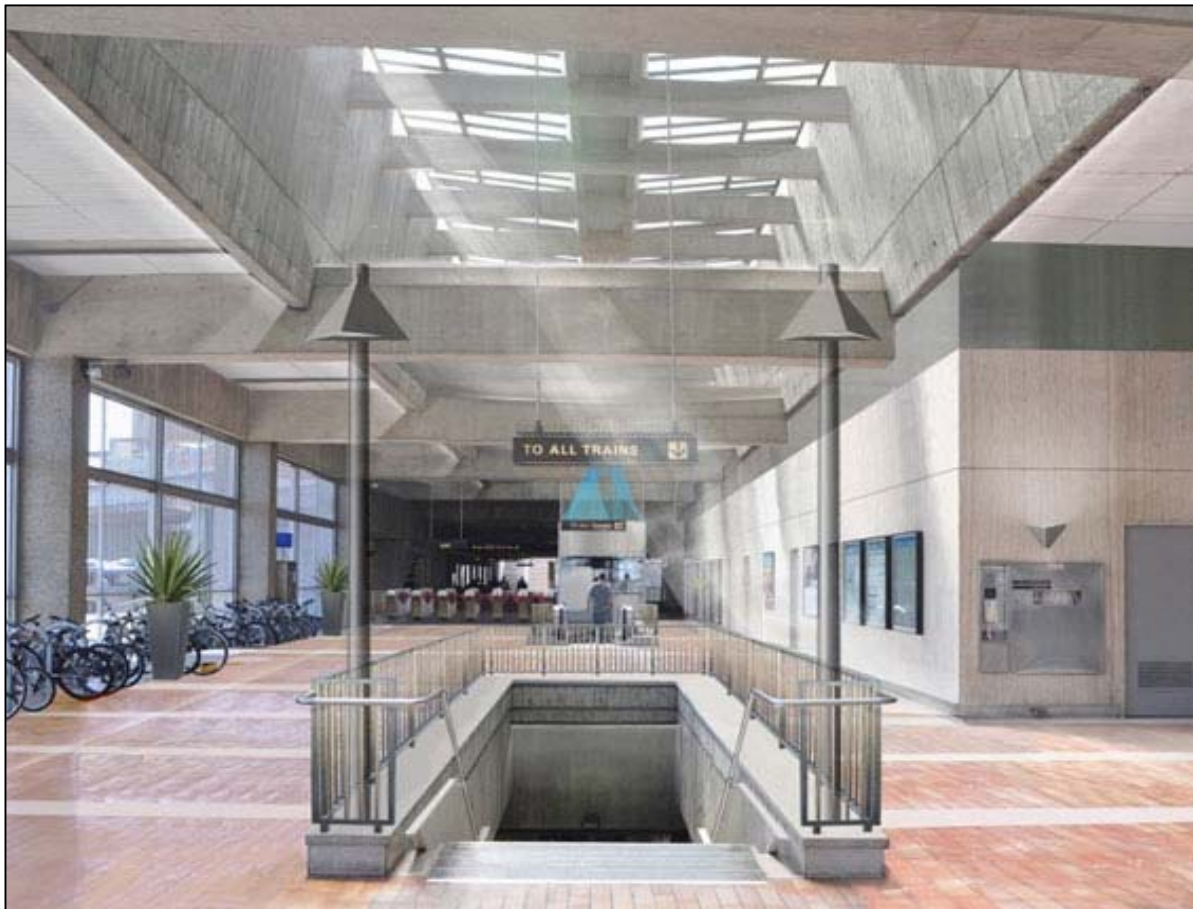
Station interior with retrofitted glass clerestory windows (included in Option #3)
