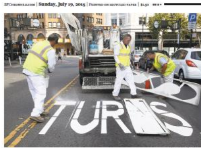
Above: Municipal Transportation Agency workers paint directions for drivers on Sixth Street as part of the Vision Zero traffic plan. Below: Areas along the curb was "daylighted" at Sixth and Howard as part of the Vision Zero traffic plan.
